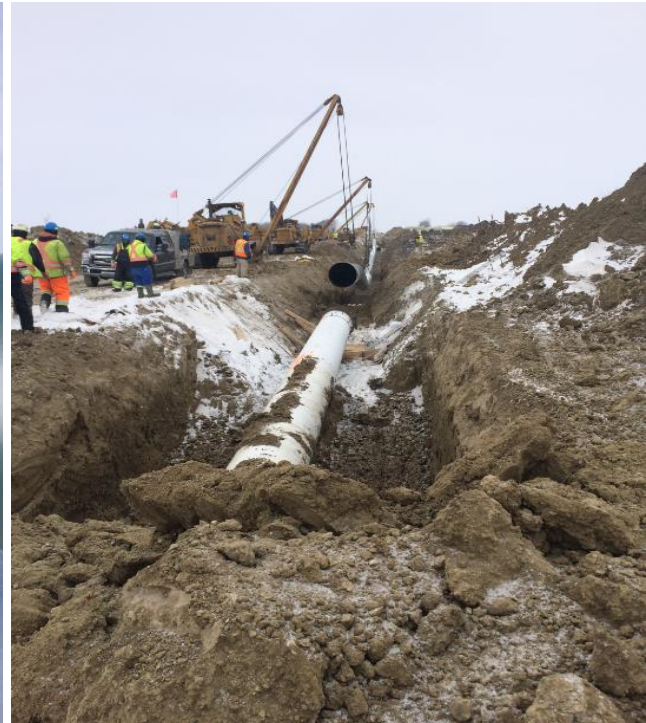
755 + 100 lowering in pipe for tie in
