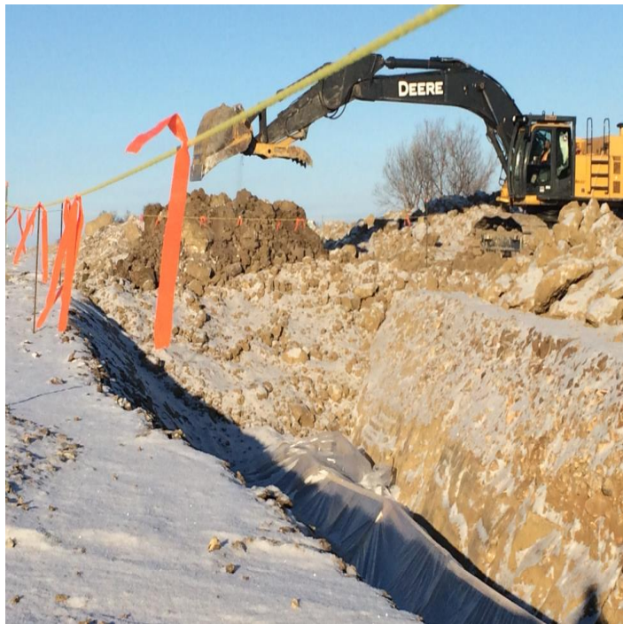
8055 + 100 backfilling ditch & pipe hoarded in
