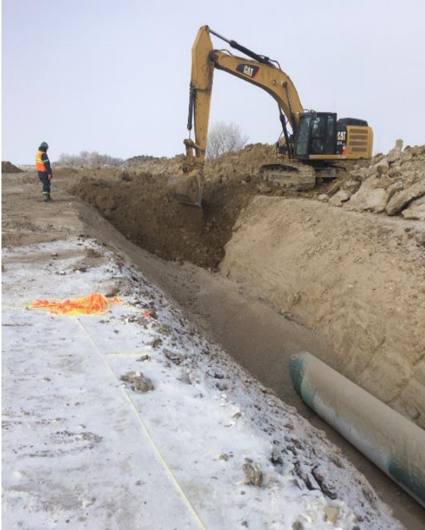
804 + 600 sand shading pipe
