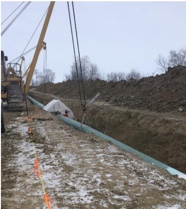
802 + 300 Welders completing tie in on pipe
