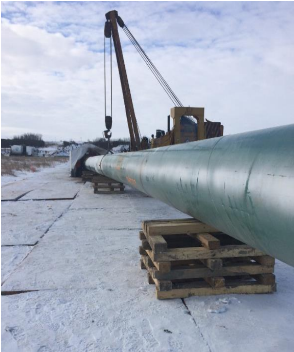
806 + 200 welding onto section
