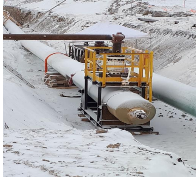
735 + 600 Hydrostatic testing head installed for testing
