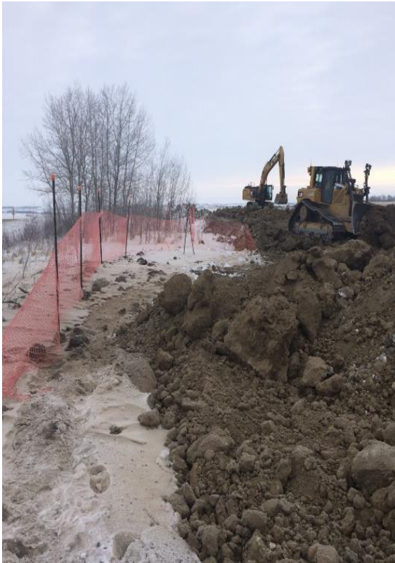
802 + 500 backfilling ditch.
